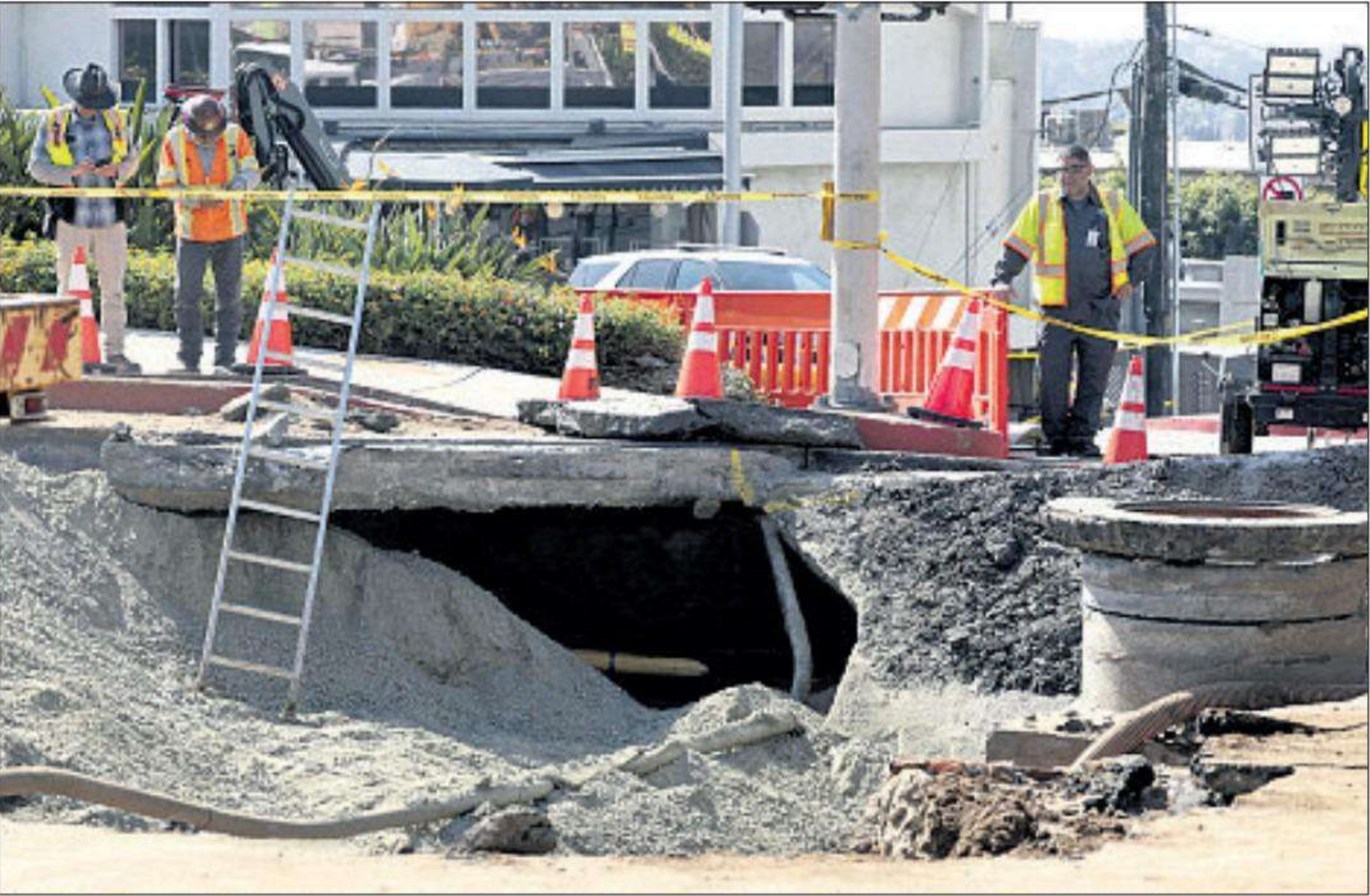
REPAIR work is underway after a severed trunk line flooded streets and shut a portion of Sunset Boulevard. MYUNG J. CHUN Los Angeles Times
