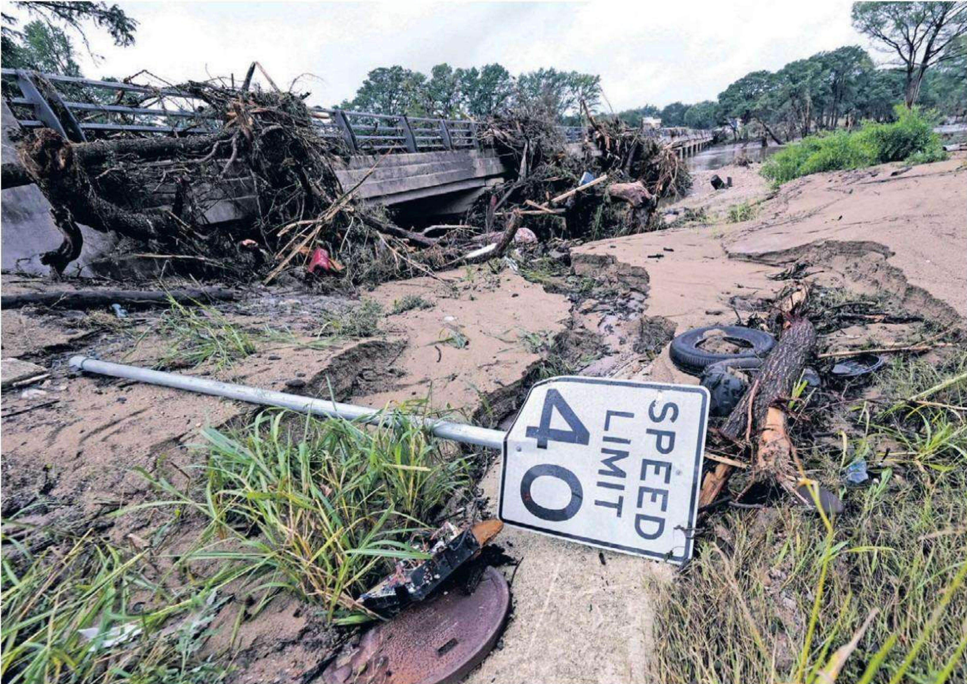
WASHOUT: Debris is left behind Friday along the Guadalupe River in Kerrville after heavy rains triggered more flooding in Texas Hill Country. At least two people have died, and first responders were rushing to help others trapped in high waters. A6
